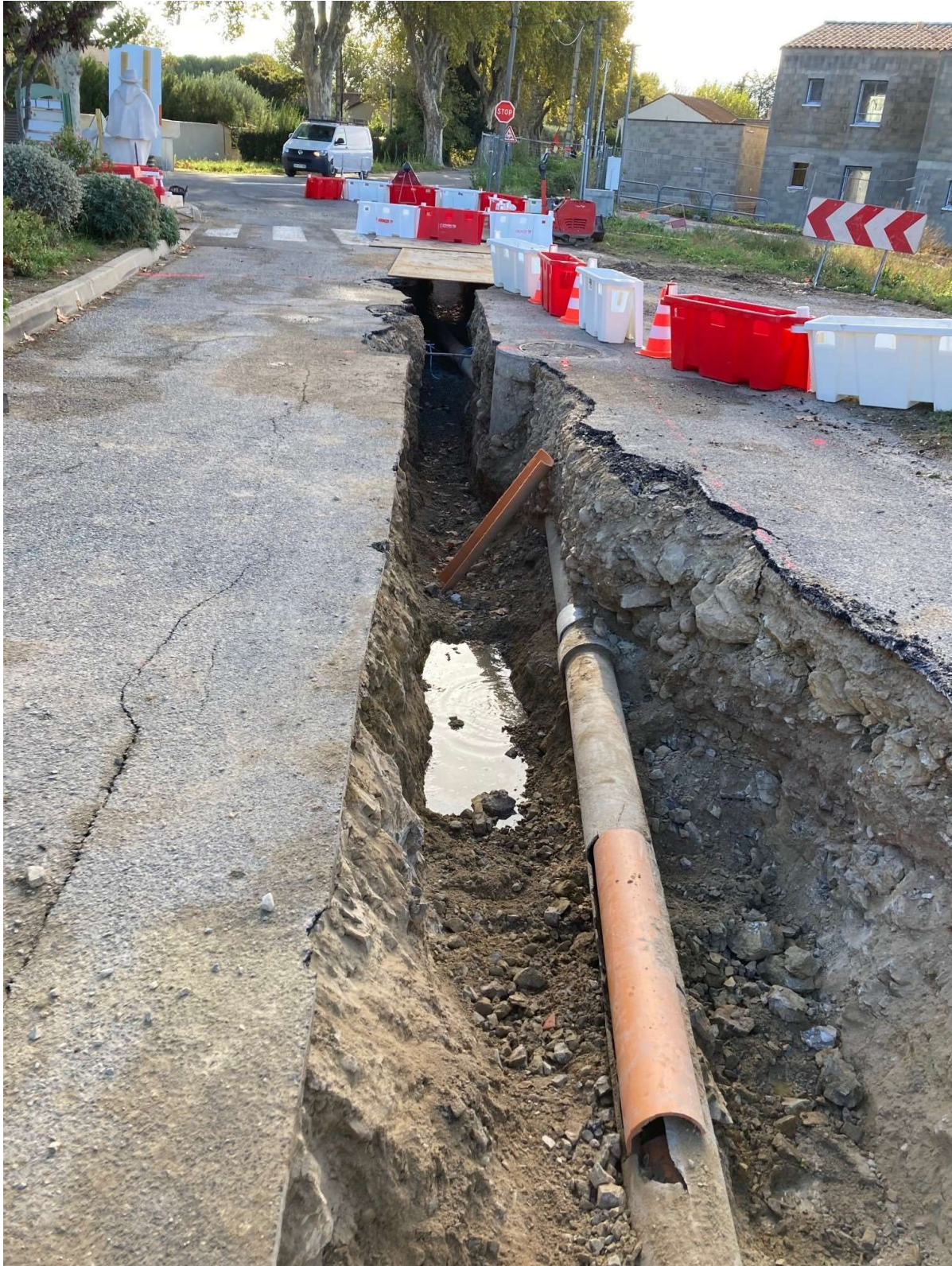
Route de Servanes - Mourières
